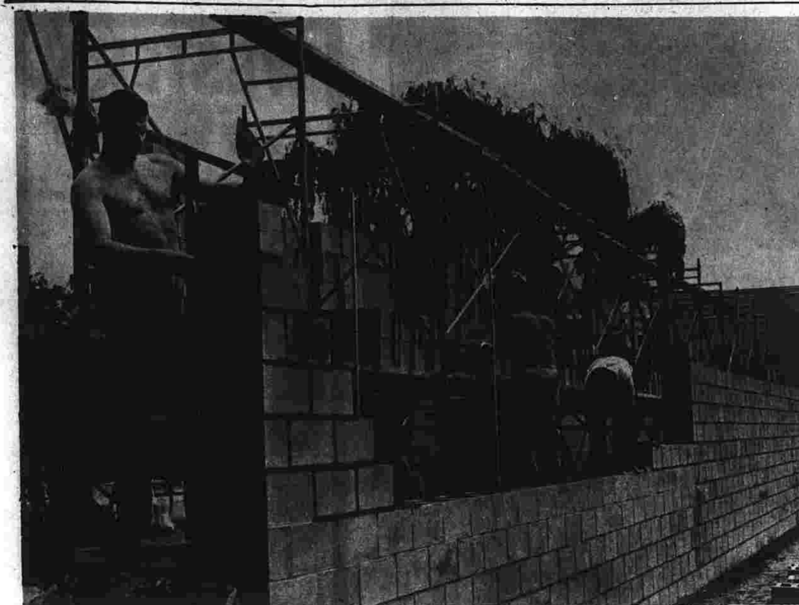
Walls Rise at New Home for The Herald
